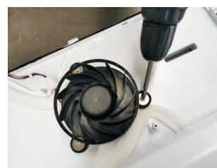
7. Removing the freezing fan
