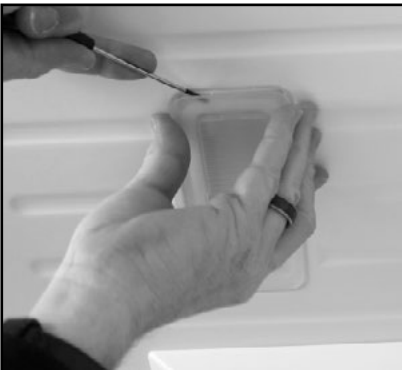
1. Unclip the lens from the ceiling to access the top light board.
