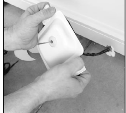
9. Unclip the fan housing and open it up.
